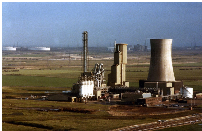
Figure 4. The ICI 'Pruteen' plant at Billingham on Teesside, UK. The specially developed airlift fermenter is the middle tower; the others are for the production of growth medium and for cooling.
